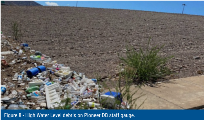
Figure 8 - High Water Level debris on Pioneer DB staff gauge.
