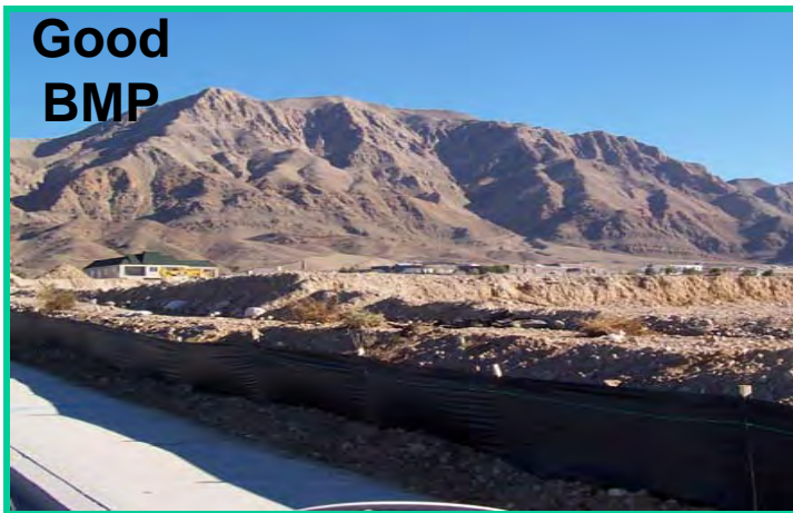
Effective, but fence installed backwards
