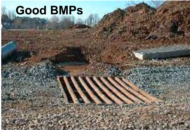
Gravel pads, tire wash areas minimize trackout
