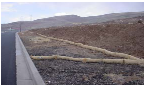
Straw waddles used for flow dissipation and erosion control. (Reno, Nevada)
