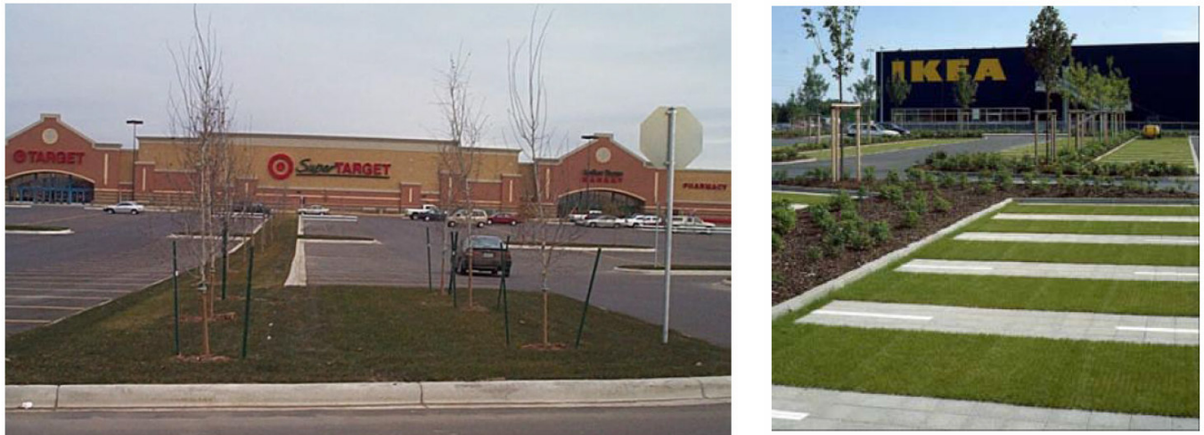
Figure 5. Comparison of Typical Parking Lot and LID Parking Lot
