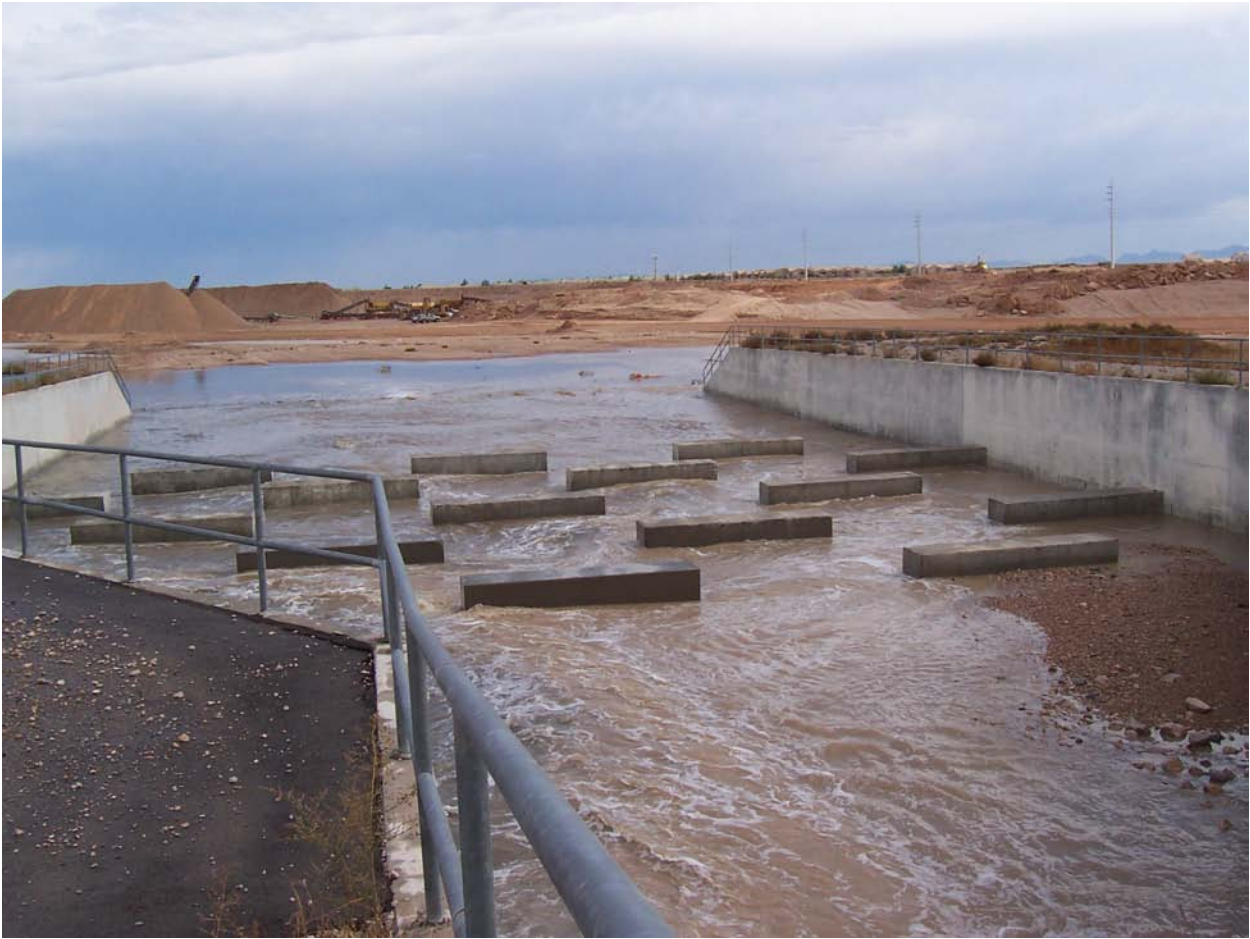
Figure 2. Upper Flamingo Detention Basin
