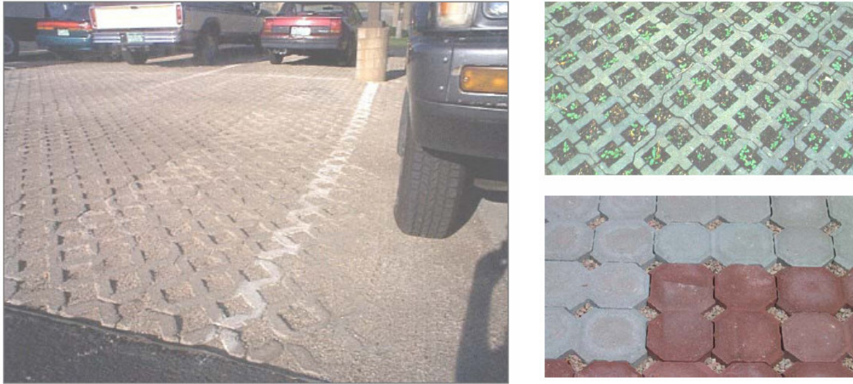
Figure 9. Porous Pavement Examples
