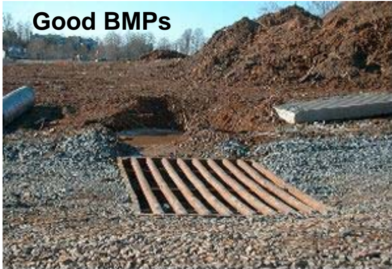
Gravel pads, tire wash areas minimize trackout
