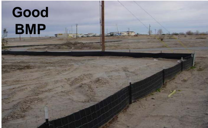
Properly installed fence
