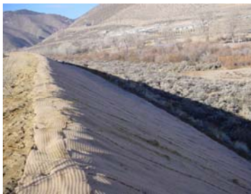
Erosion Control Fiber Matting (Carson City, Nevada)
