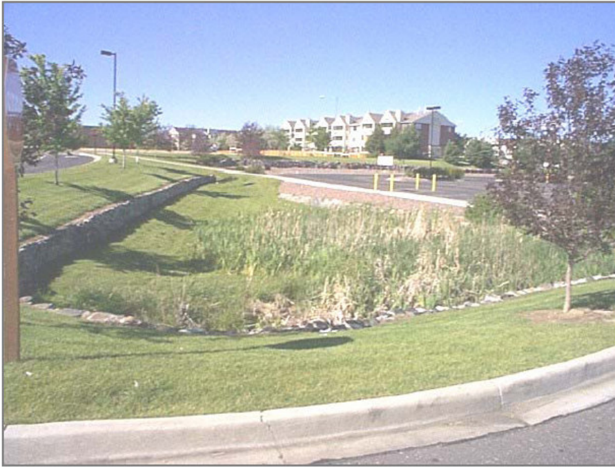
Figure 7. Extended Detention Basin Example
