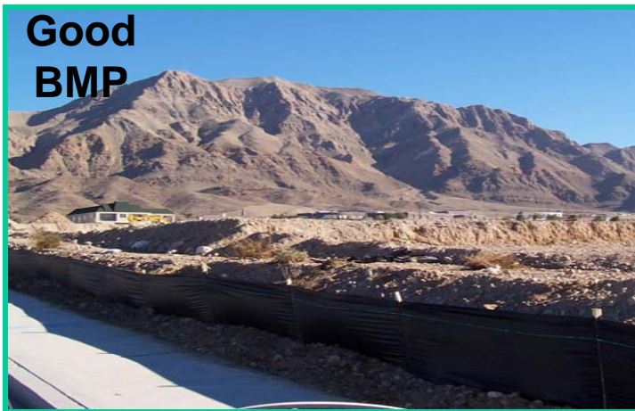
Effective, but fence installed backwards
