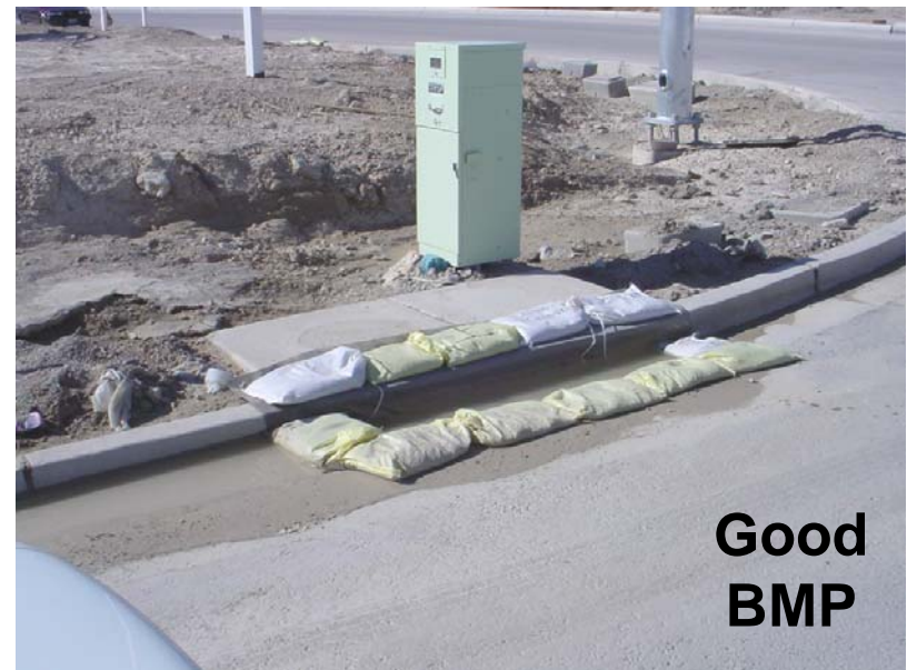
Effective use of gravel bag BMP
