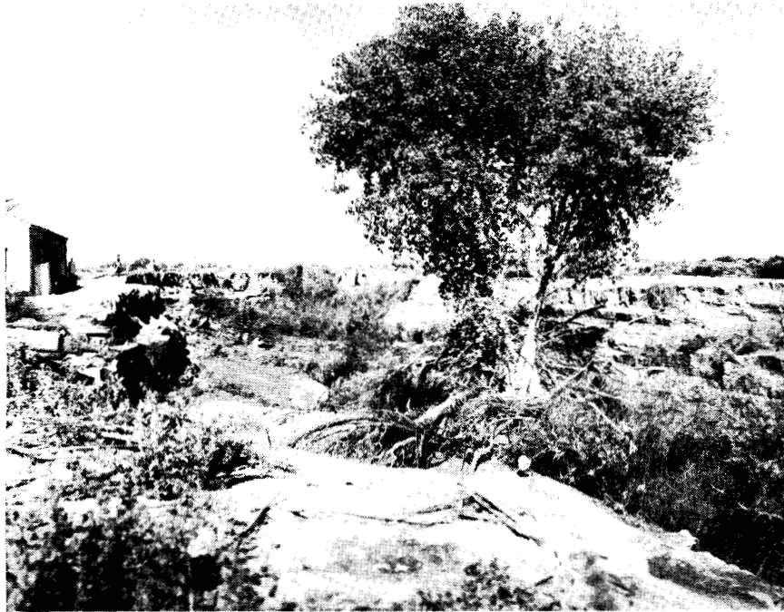
Figure 14 — Flood of 1960 along the Muddy River resulted in eroded banks and a large amount of debris piled against a tree. The debris reflects the depth of water during the flood. The site is about 3 miles north of Overton.
