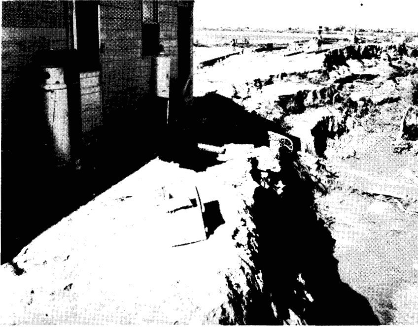
Figure 15 — A closeup view of bank erosion damage shown in Fig. 14.
