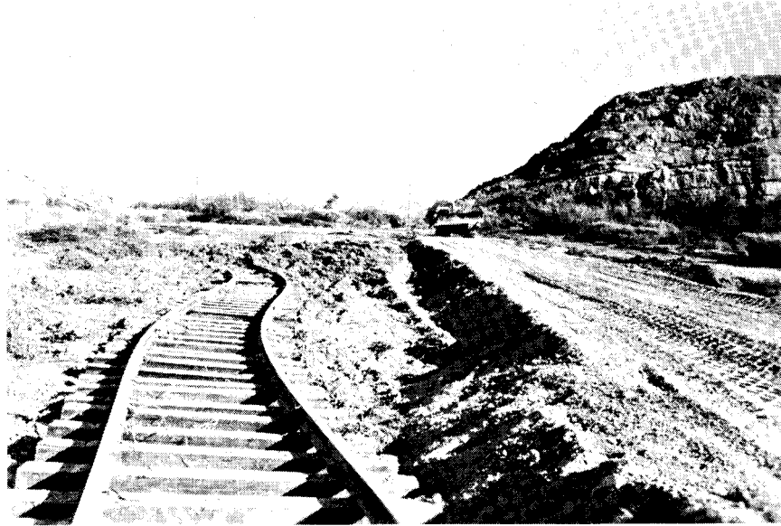
Figure 6 — Railroad damage due to flooding in the Narrows between upstream limit of study and Glendale during the flood of 1960.
