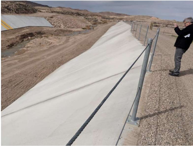
On east bank facing upstream at approximately between HEC-RAS Station 2135.97 and 1434.90.
