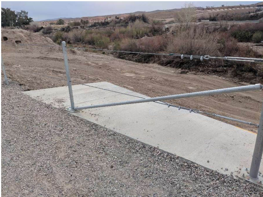
East bank facing downstream at approximately HEC-RAS station 710.16.
