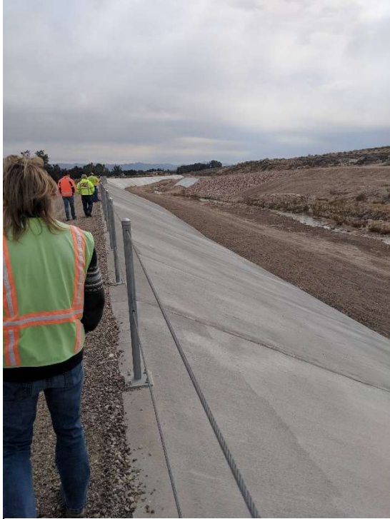
On east bank facing downstream at approximately HEC-RAS Station 2824.16.
