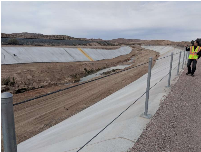
On east bank facing upstream just upstream of approximately HEC-RAS station 1434.90.
