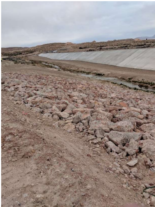
On west bank facing upstream at approximately HEC-RAS station 2191.11.
