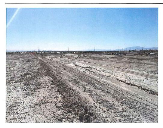
Facing south. Graded earthen channel south of the 12x6 arch culvert outlet.
