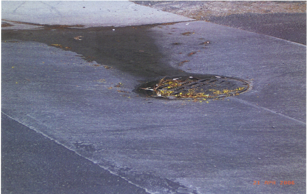
Picture 7. Area inlet located within a valley gutter at the intersection of Burnham Avenue and Sur Este Avenue.
