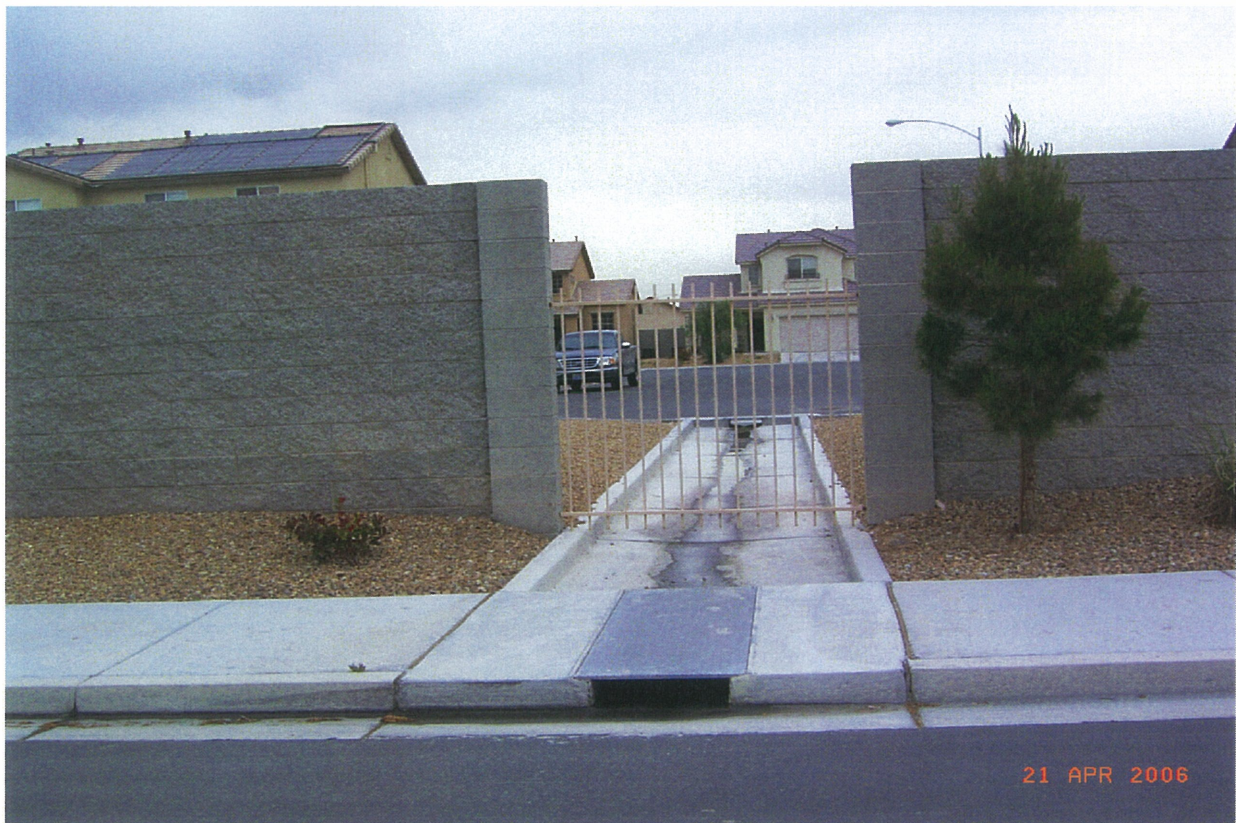
Picture 5. 5' drainage easement that drains flow from Basin ROB8 to Burnham Avenue.
