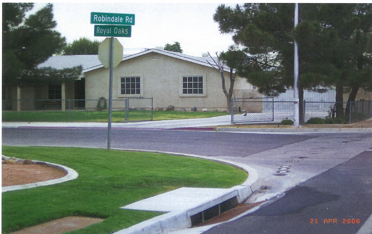
Picture 3. 5' drop inlet at southeast corner of Robindale Road and Royal Oaks.
