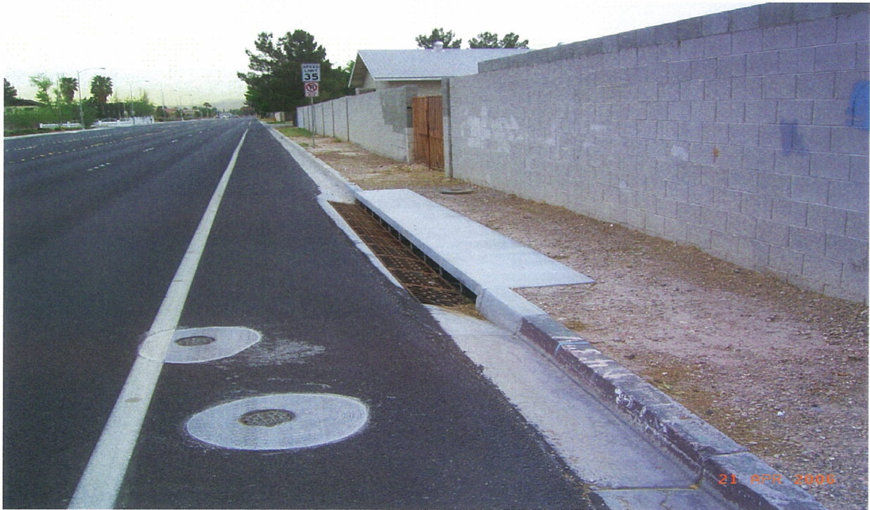
Picture 1. 15' drop inlet on south side of Robindale Road (approximately 150' east of Branding Iron Lane).
