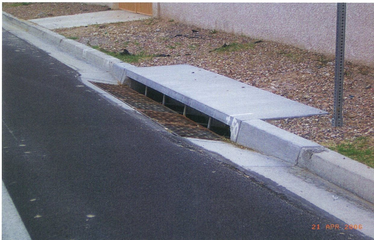
Picture 4. 7.5' drop inlet located approximately 100 feet east of drop inlet in Picture 3 above.
