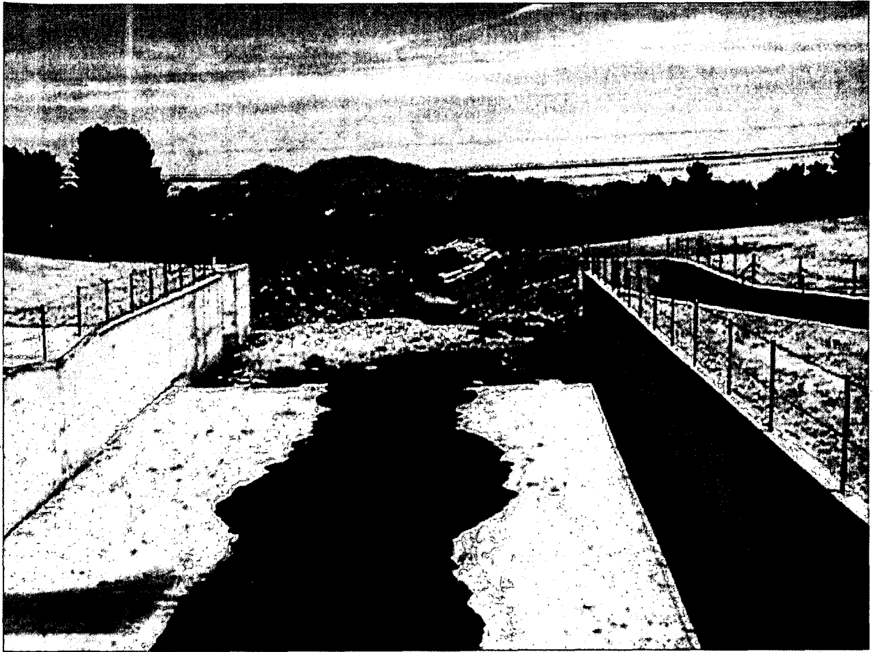
Photo 1 - Energy Dissipator and End of Concrete Channel Downstream of Spencer Street
