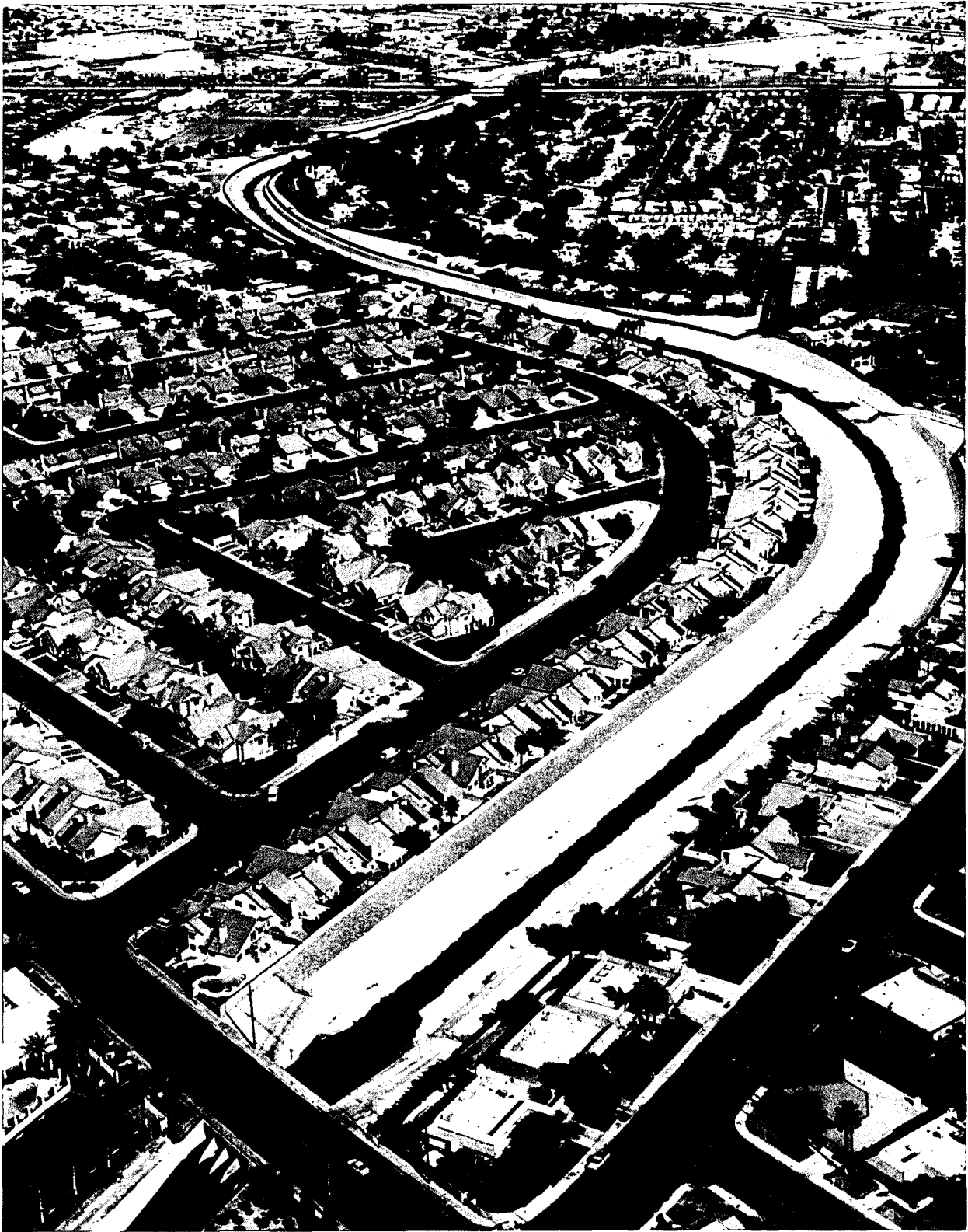
Photo 1 - Flamingo Wash Improvements from Mojave Road to Boulder Highway looking downstream towards Boulder Highway. Mojave Road is located in the lower right hand corner of the photo and Boulder Highway is across the top of the photo.
