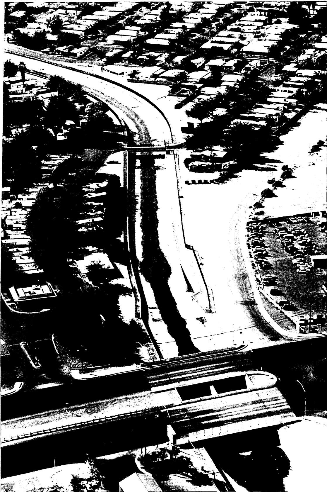
Photo 2 - Flamingo Wash Improvements looking upstream of Boulder Highway.
