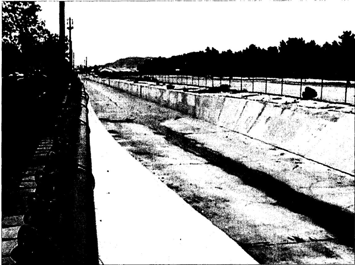
Photo 2: Gowan Outfall looking downstream at the transition to a rectangular channel.
