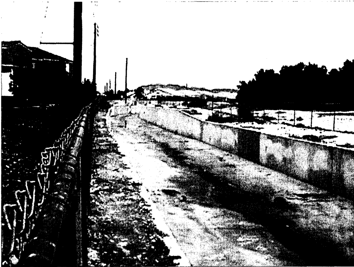
Photo 3: Gowanus Outfall looking downstream at the transition from a 30' wide channel to a 25' wide channel.
