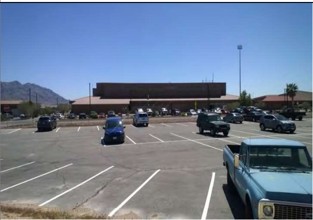
Photo 6: View from North Site looking South.
