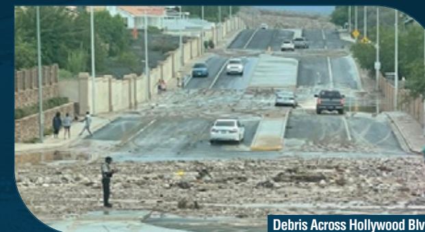
Debris Across Hollywood Blvd.
