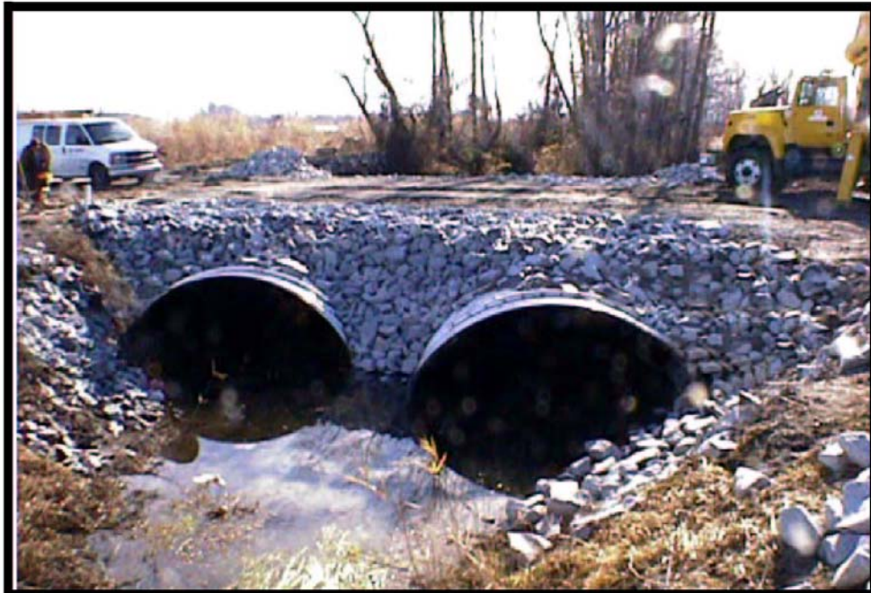
Temporary access culvert (Courtesy of NCDOT)
