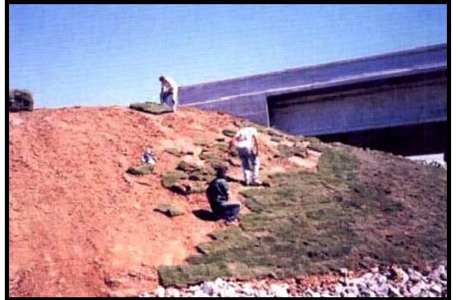
Applying sod to a slope (Courtesy of Douglas County)
