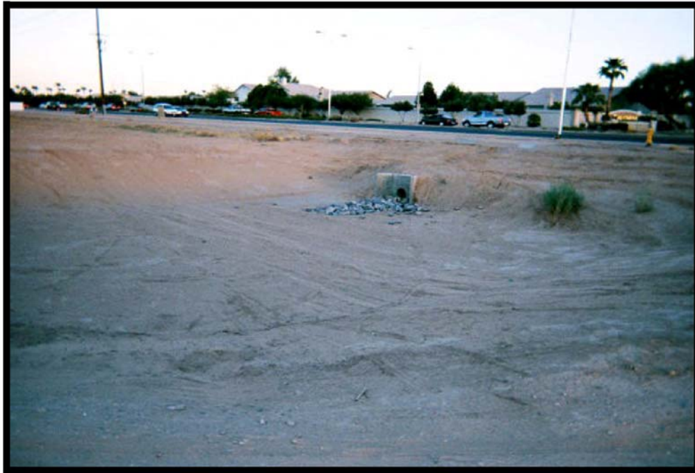
Temporary sediment basin with outlet protection (Courtesy of Maricopa County)
