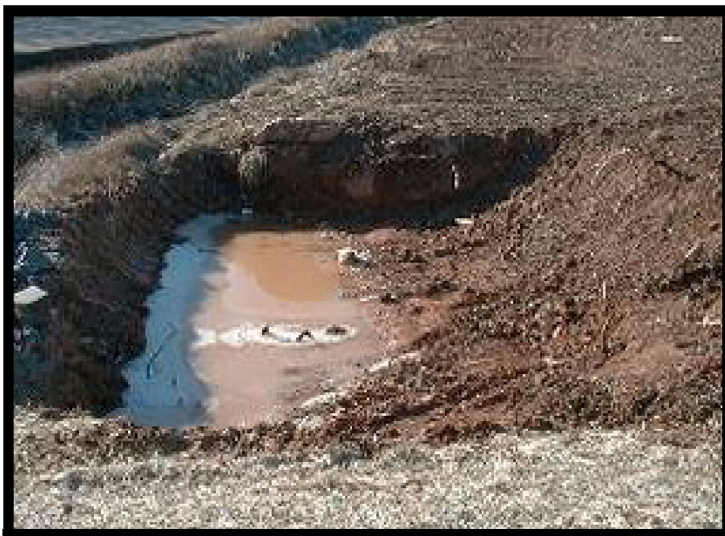
Sediment traps are used to collect sediment laden runoff from disturbed areas on construction sites (Courtesy of Douglas County)
