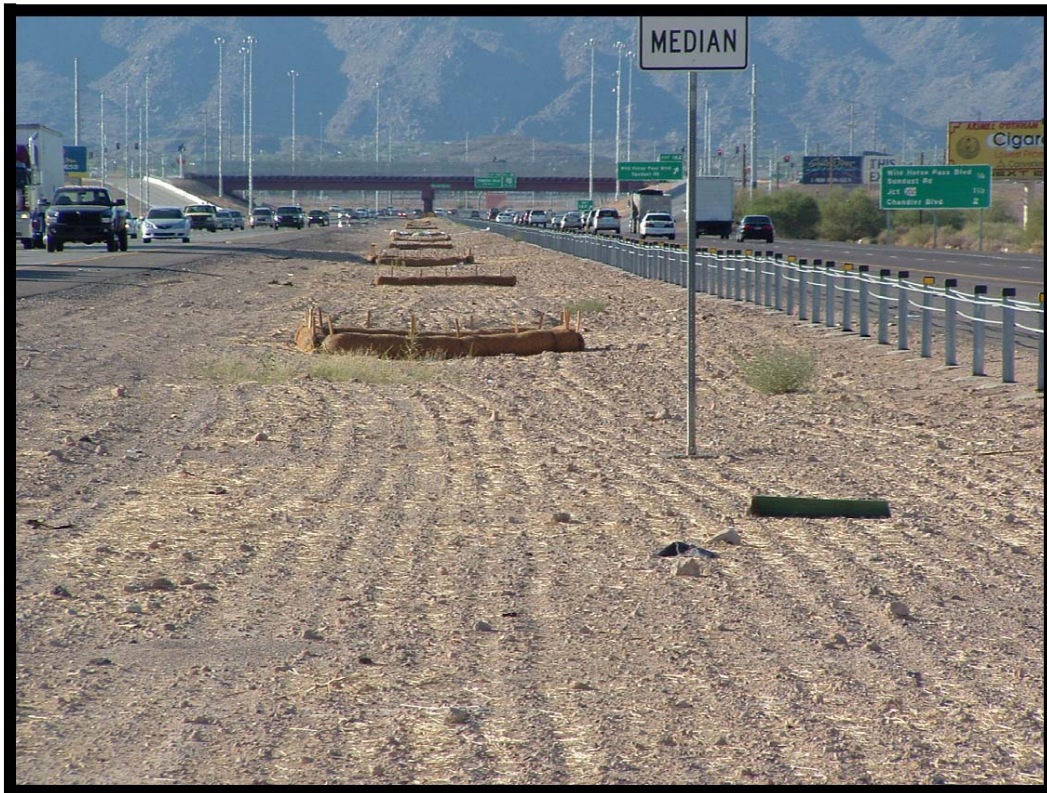
Use of an organic filter barrier in the highway median (Courtesy of Maricopa County)
