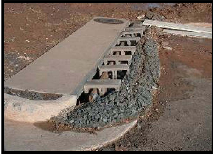
Straw wattle inlet drain protection (Courtesy of Douglas County)
