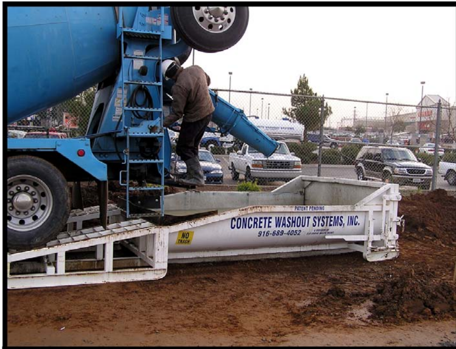
Concrete washout area (Courtesy of Douglas County)
