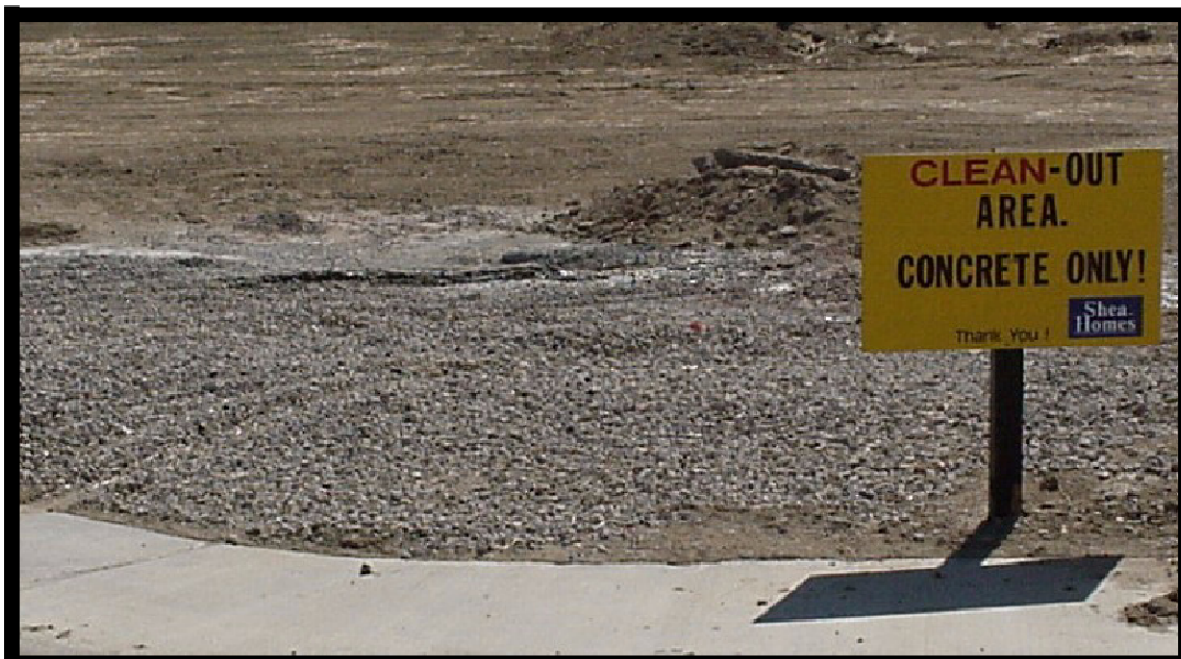
Concrete washout area (Courtesy of Douglas County)
