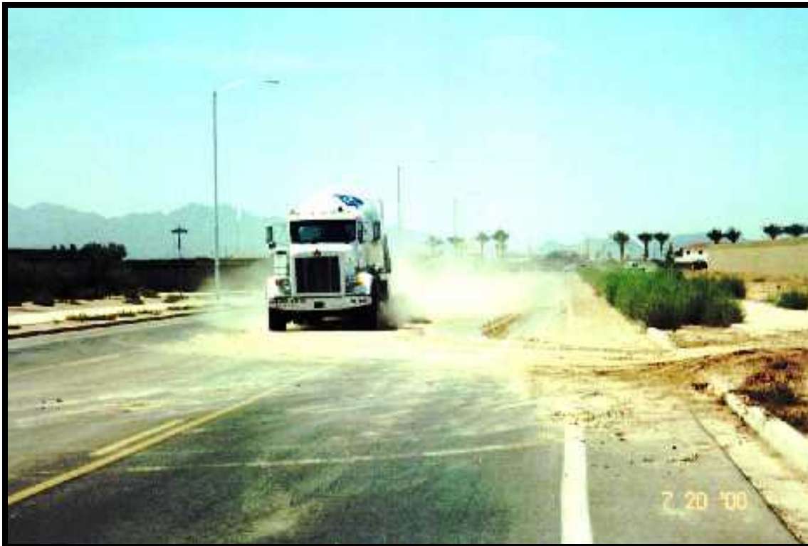
Construction site trackout (Courtesy of Maricopa County)
