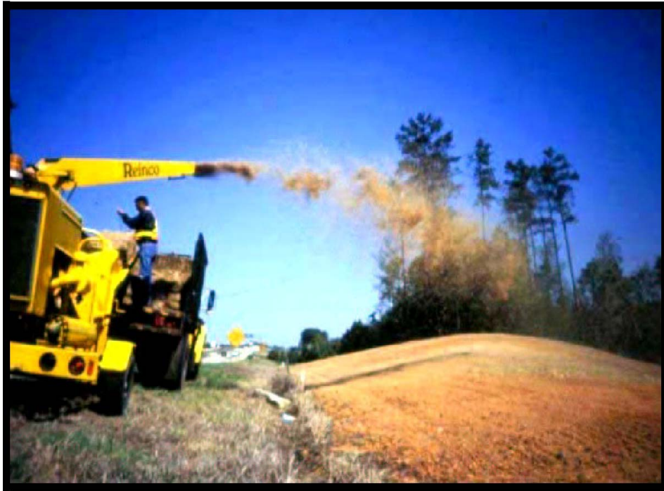
Mechanical chipper application of mulching (Courtesy of NCDOT)
