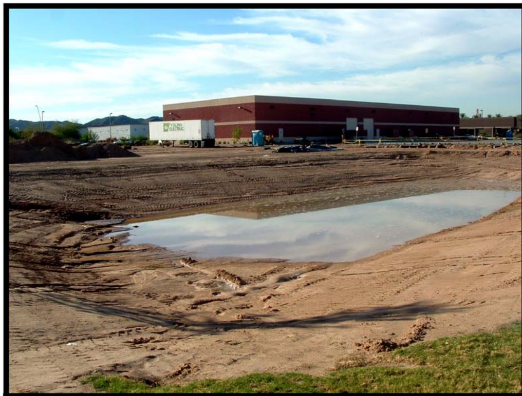
Temporary sediment basins provide stormwater storage during the construction process (Courtesy of Maricopa County)
