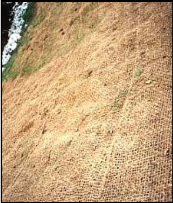
Biodegradable erosion control (Courtesy of EPA)
