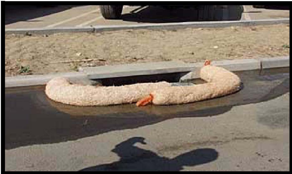
Straw wattle inlet drain protection (Courtesy of Douglas County)
