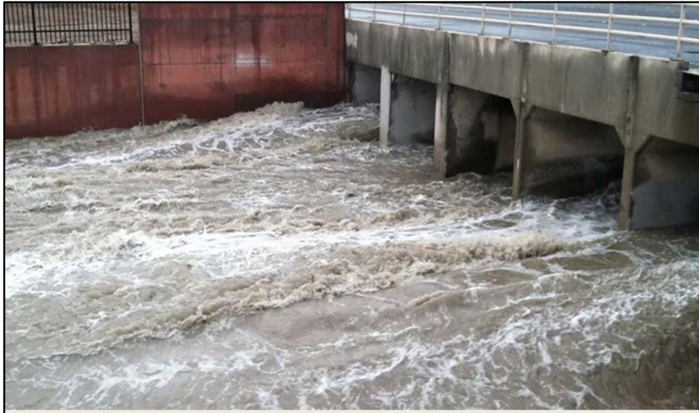
Flamingo Wash at Eastern Avenue
