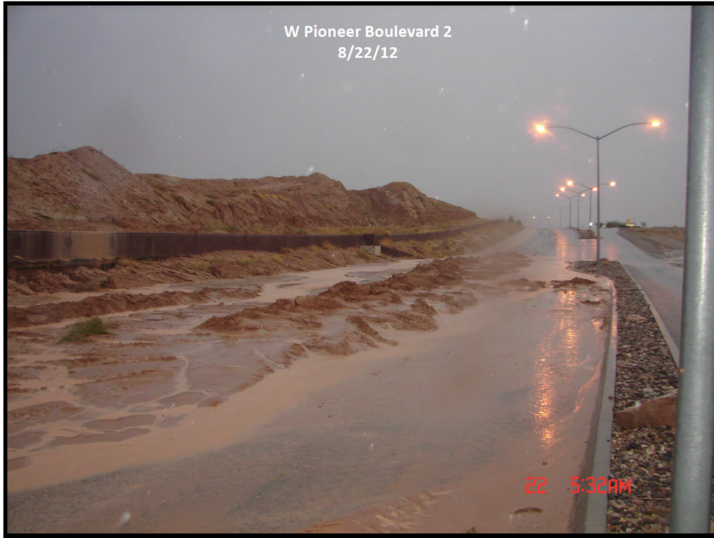
And clean-up of soils in the roadways.
