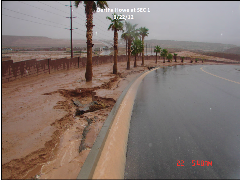
Damages in Mesquite were mostly limited to erosion of landscaped areas...
