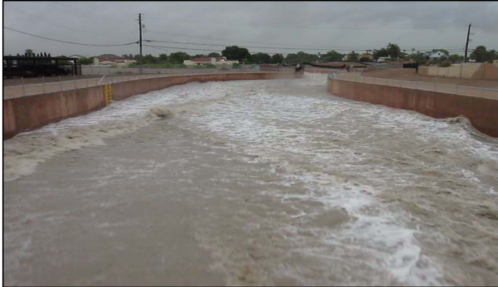
Flamingo Wash at Eastern Avenue
